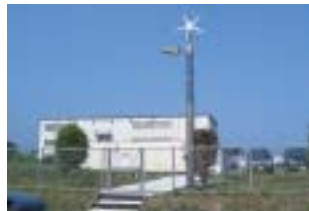
Hybrid light using solar light and force of wind Silicon solar cell: 96 W Wind power generation: 50 W
