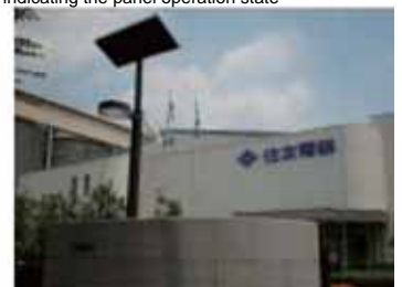
Solar panels at Sayama site and light
