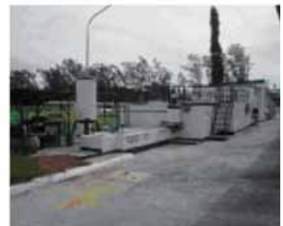
Wastewater treatment facility (capacity: 220 t / day)
