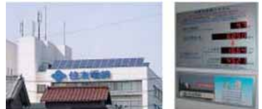
Solar panels on the roof of the headquarters building, and a board indicating the panel operation state
