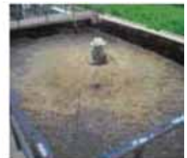
Aeration tank for wastewater treatment
