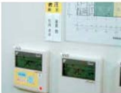
Timers on air conditioners automatically turn them off when not necessary.
