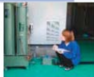
Compressor drain check
