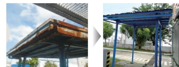
Before (left) and after (right) repair
