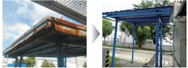
Before (left) and after (right) repair
